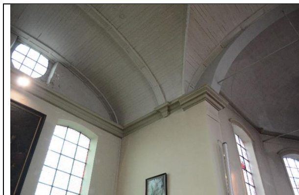
Plafond N-transept © M in O.
