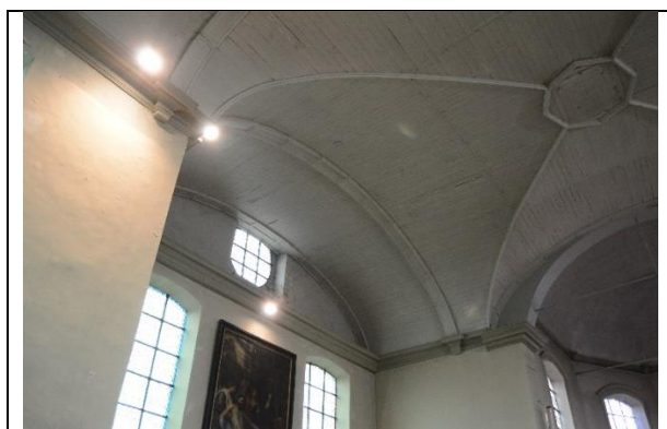
Plafond N-transept © M in O.
