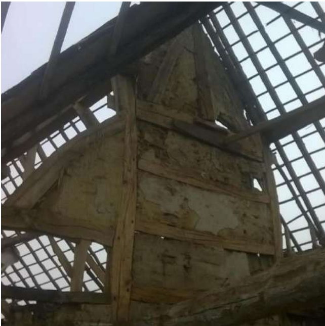
Afb. 73: Origineel eindspant op as 6.
