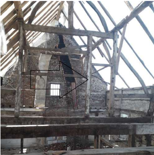
Afb. 55: Deuropening dakspant as 3
