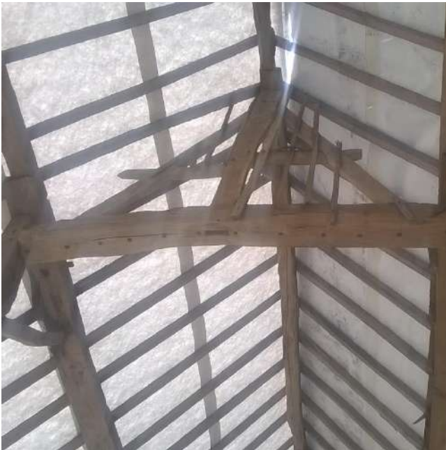
Afb. 85: Restanten pannen beschieting as 3.
