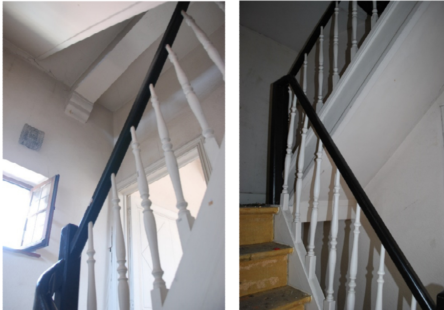
Afb. 142: Detail traphal verdieping.
