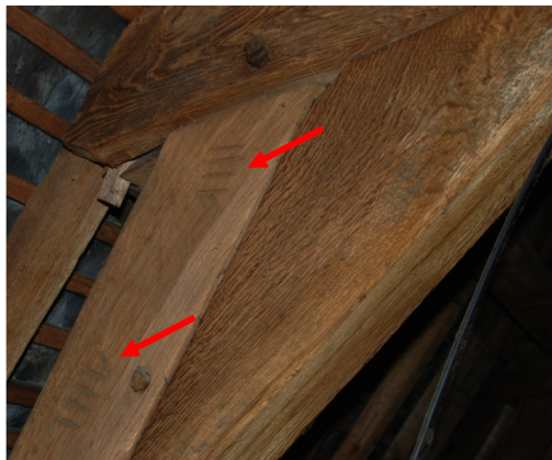
Afb. 163: Detail zolder – dakgebinte -IIII.
