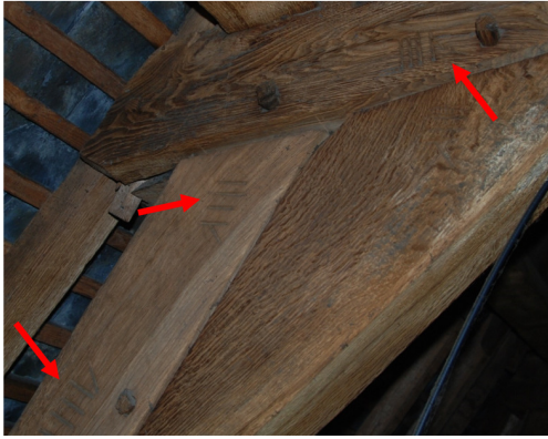
Afb. 162: Detail zolder – dakgebinte -IIII.
