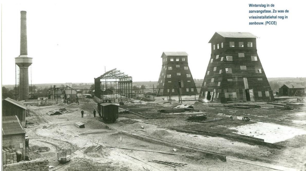
Figuur 3: De houten afdiepingstorens. © PCCE
