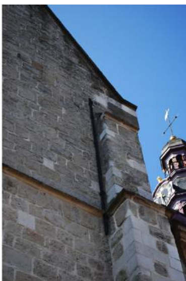
muuranker steunbeer transept
