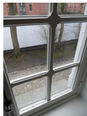
52A – verdieping enkele beglazing
