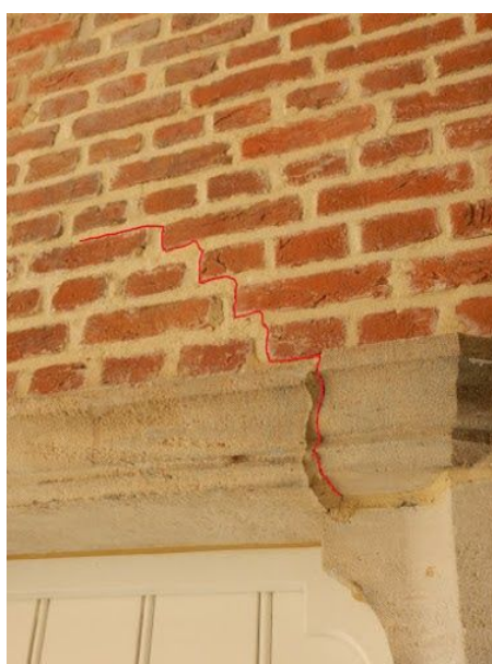
[16]-west: scheurvorming boven deur
