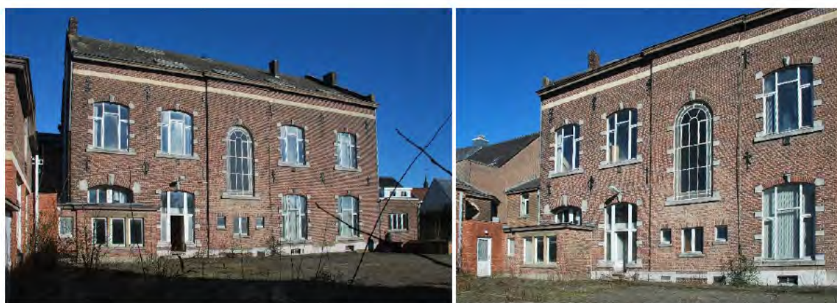
Afb. 13 achtergevel ©Studiebureau Monumentenzorg (d.d. 15/02/2019)
