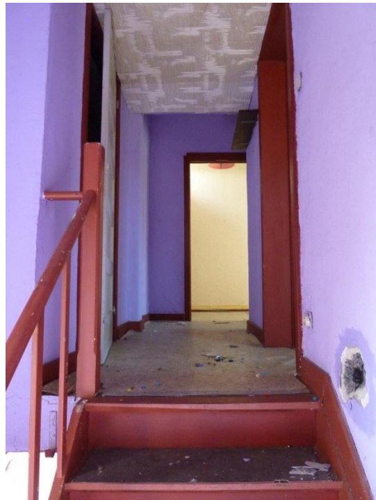
Foto 32: woning 16: hal verdieping
