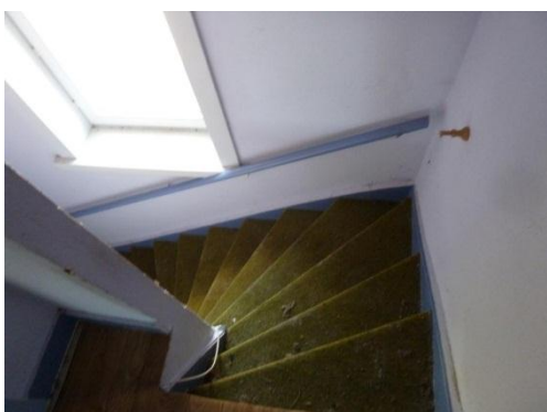
Foto 51: woning 4: trap verdieping
