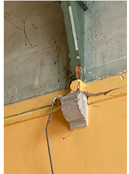
Afb. 135. – Detail hardstenen console
