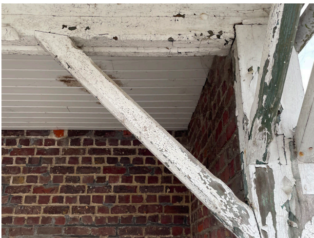
Afb. 86. – Detail dakoversteek in houten cottigestijl
