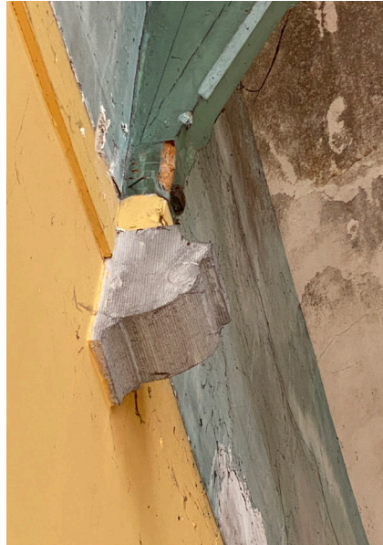
Afb. 131. – Detail hardstenen console
