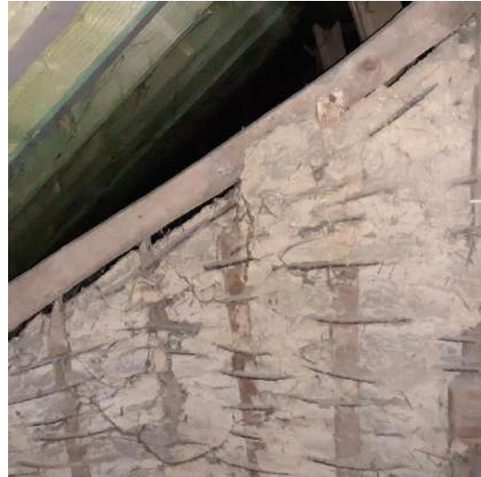
Afb. 115: Kempens vitswerk spant as 4.
