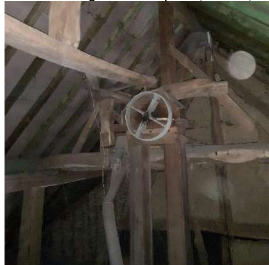
Afb. 117: Spant as 5 met elevator.
