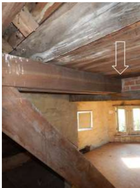
Oplegging dekbalk spant zolder [2]
