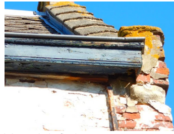
bakgoot-schade afkasting
