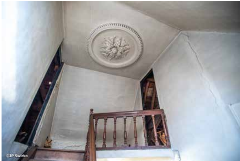
Rosette boven bordes zolderverdieping.
