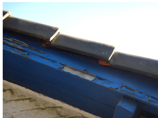
dak [1]-west: dakrand
