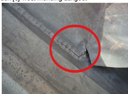
dak [3]-noord monding zakgoot
