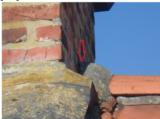
Losgescheurde mortelaanwerking.
