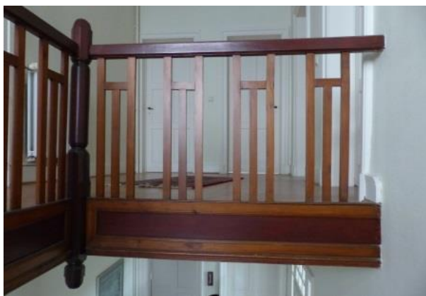
Figuur 138 Detail balustrade (AS, 13.02.2019)
