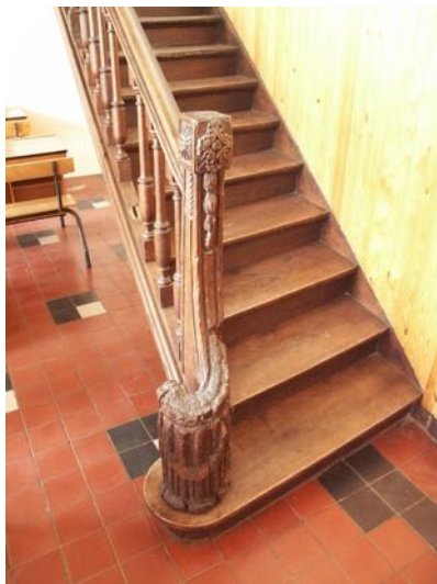
Monumentale trap in pand A
